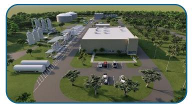
The water production facility is a reverse osmosis (RO) water treatment facility currently under design. RO is widely regarded as the leading water purification technology in the water treatment industry. It removes unwanted sediments and salts by filtering water through "semi-permeable membranes" and capturing them at the molecular level, leaving behind high quality, great tasting drinking water. Water from the production facility will be piped directly to member government utilities.
