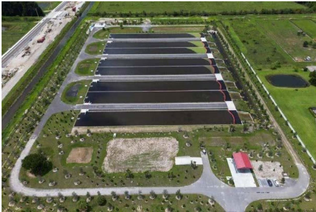
The St. Johns River Water Management District (SJRWMD) opened the Moorhen Marsh Low Energy Aquatic Plant System (LEAPS) stormwater treatment facility earlier this year. The facility pulls in 10 million gallons of water per day from the North Relief Canal and diverts it to the Moorhen Marsh site to be treated, ultimately helping restore the Indian River Lagoon. (Photo: SJRWMD)
