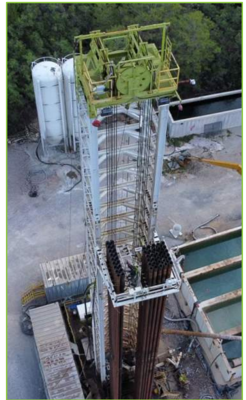
LFA deep-well drilling rig
