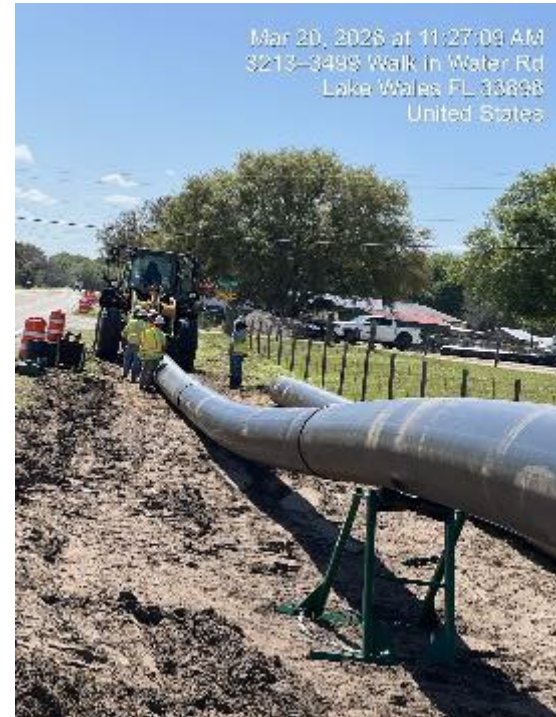
Raw Water Main Pipe Fusing Walk-in-Water Road
