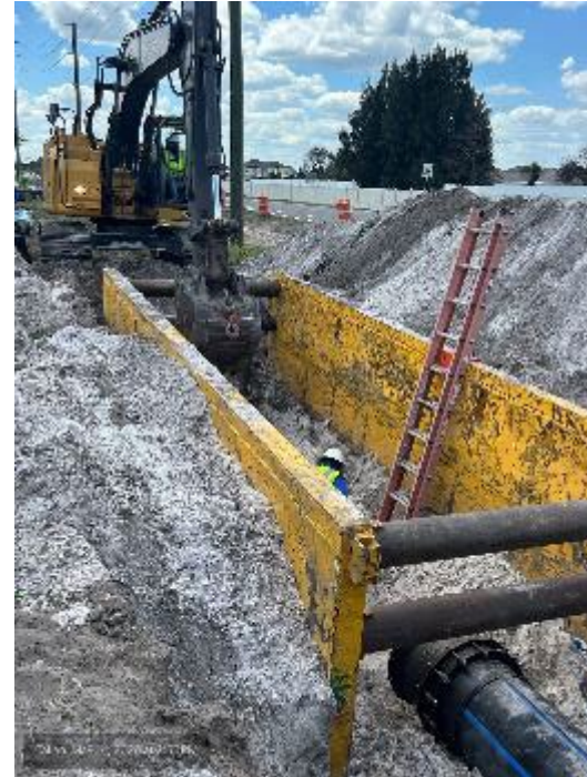
Const Package 5 24" PVC/HDPE Construction Bomber Road
