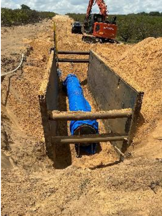
Const Package 2B 30-inch DIP Open Cut Mountain Lake Grove Road
