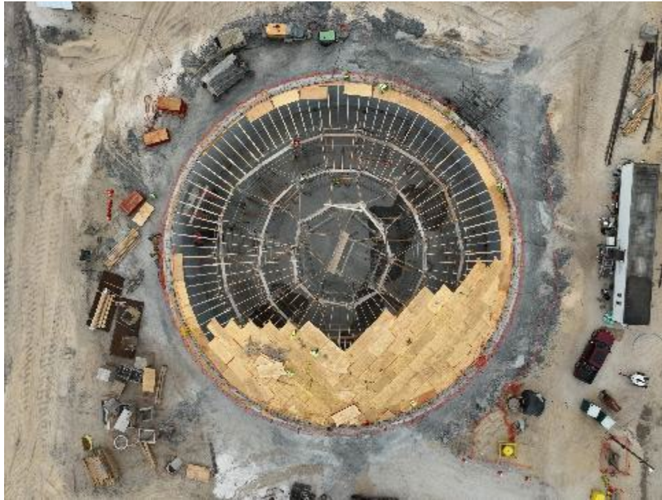
GST #1 Dome Formwork
