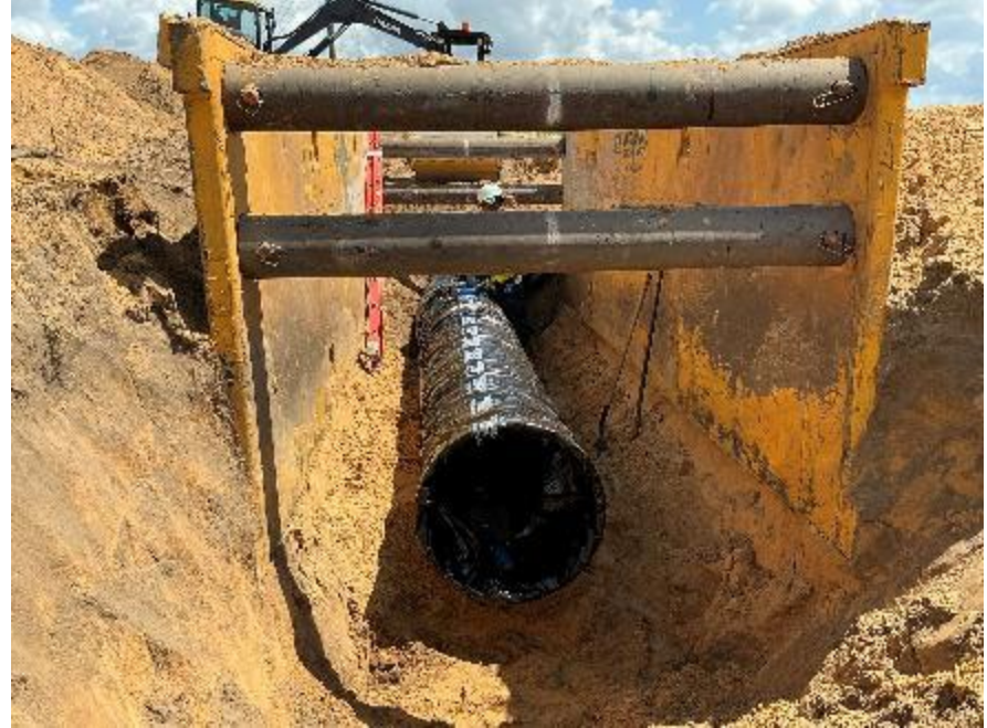
Const Package 2C 30" DIP Construction Lake Mabel Loop Road
