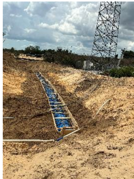
Const Package 3A Concrete Encasement for 30-inch DIP
