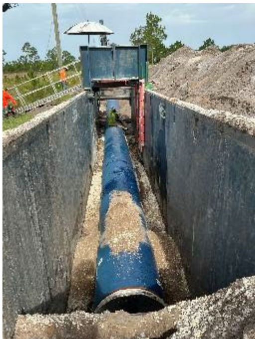
Const Package 1 42-inch Steel Pipe Open Cut Roy Keen Road
